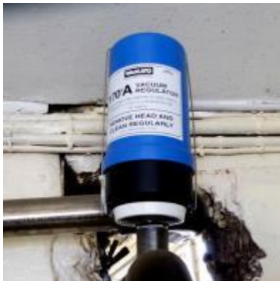
Waikato 170A regulator controls the vacuum level.
