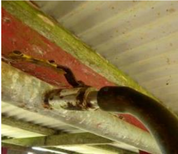
Vacuum connection to vacuum line. One could use a simple snap clamp instead of the valve.
